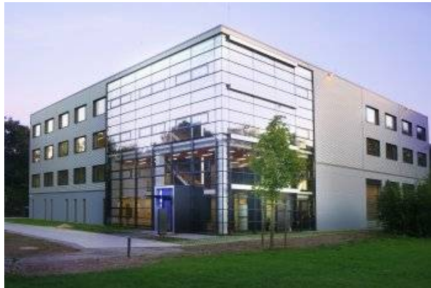
The existing building
